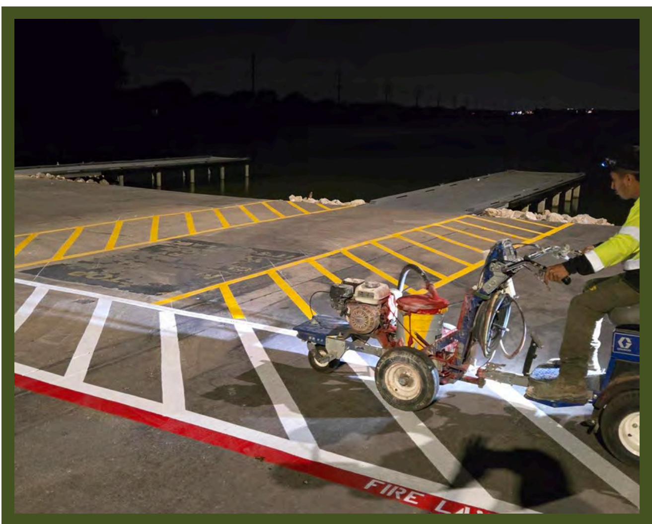
66 BOAT RAMP PARKING SPACE PAINTING
