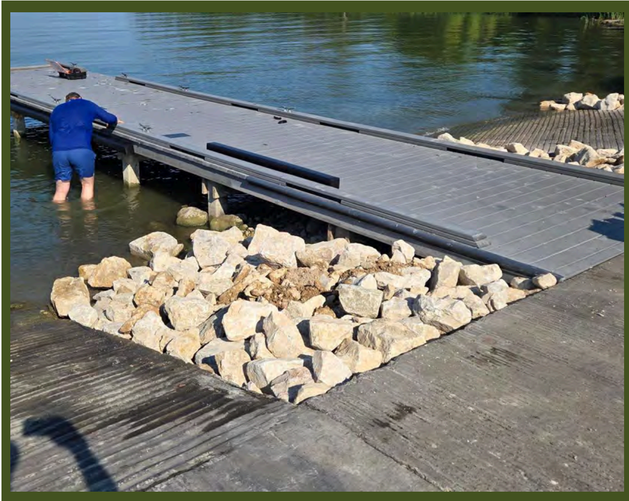
66 BOAT RAMP DOCK AND REFURBISHMENT
